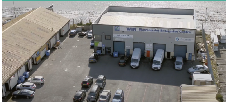
Warrenpoint Enterprise Centre, South Down
