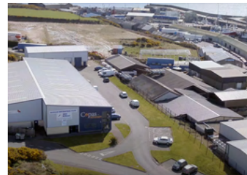
Binnian Enterprise Centre, Kilkeel, South Down
